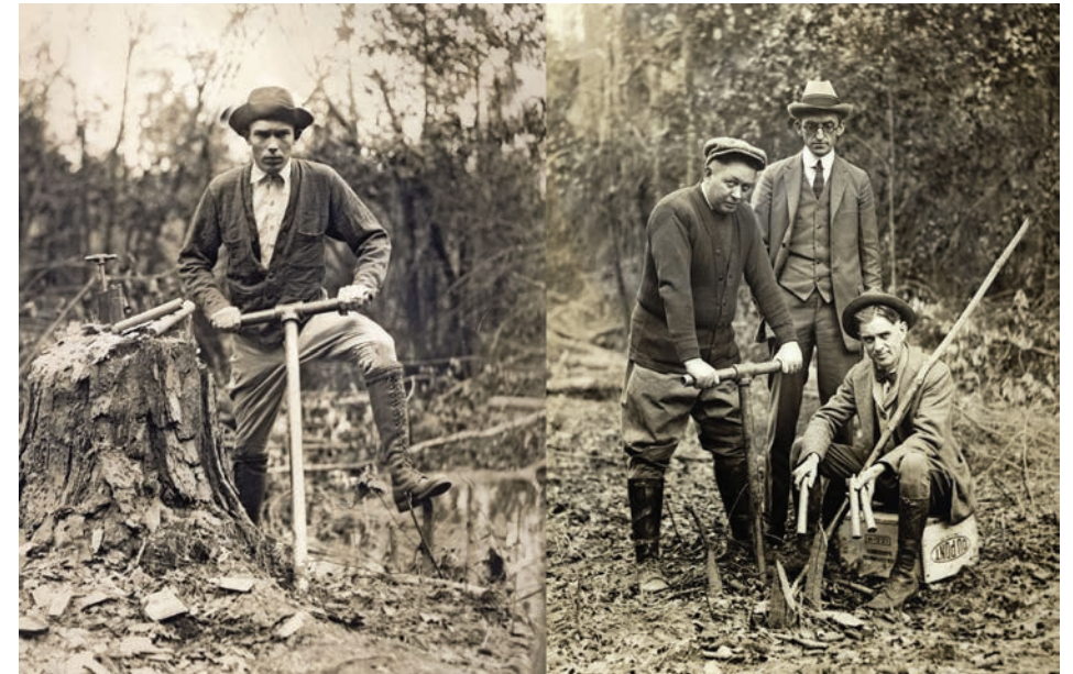
Fig. 03 In the southern United States, dynamite was a preferred tool of the military’s malaria eradication effort. Determined to eliminate any standing water bodies that might serve as a breeding ground for female Aedes aegypti , the military built drainage channels in and around their military bases to encourage the movement of water. The most expedient method of removing tree stumps from the planned drainage channels was by embedding dynamite underneath and within tree stumps, as photographed here during the 1940s or 1950s. Content provider: Centers for Disease Control. Source: https://phil.cdc.gov/phil/details.asp .
